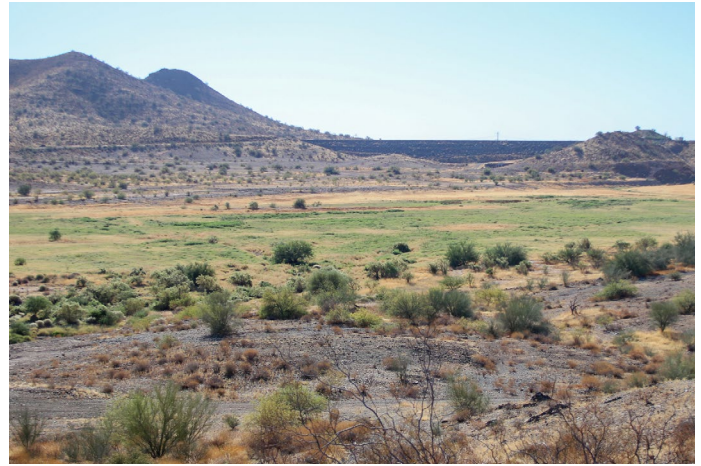
Figure 2. Basins: catchments behind dams and dikes are important sources of water following rain and dominated by invasive grasses and mesquite. This view is from the western end of Cave Creek Dam looking to the southeast over a new, rolled earth dam, Cave Buttes Dam (right) and Dike # 1 (center), 27 October 2023. Photo by R. W. Bowker
